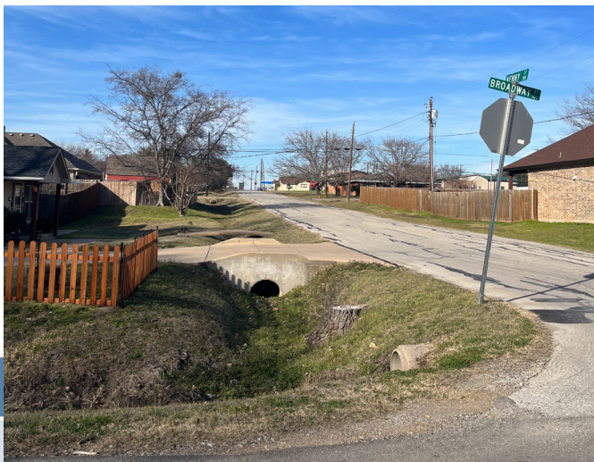
Stormwater infrastructure on a residential street.
