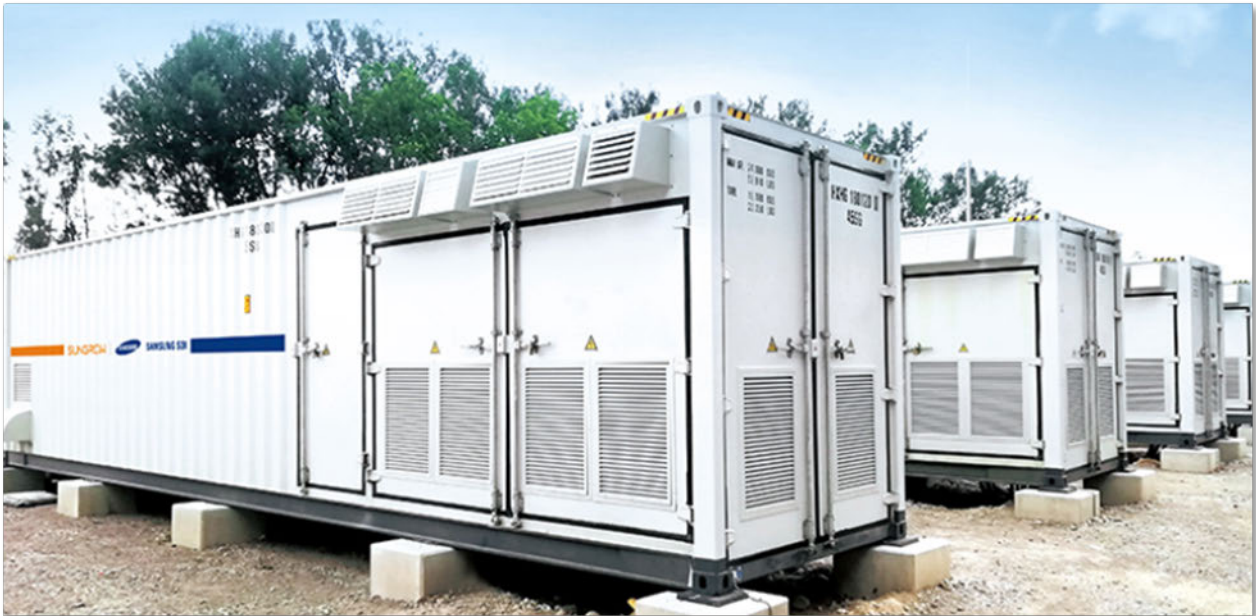
Figure 2- Battery on Pier
