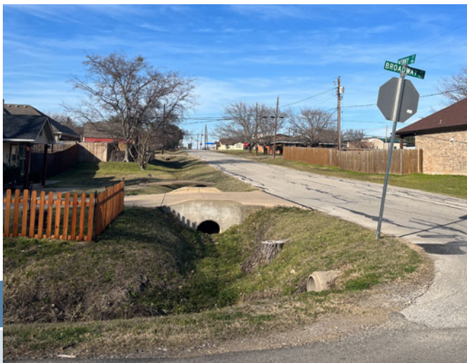
Stormwater infrastructure on a residential street.
