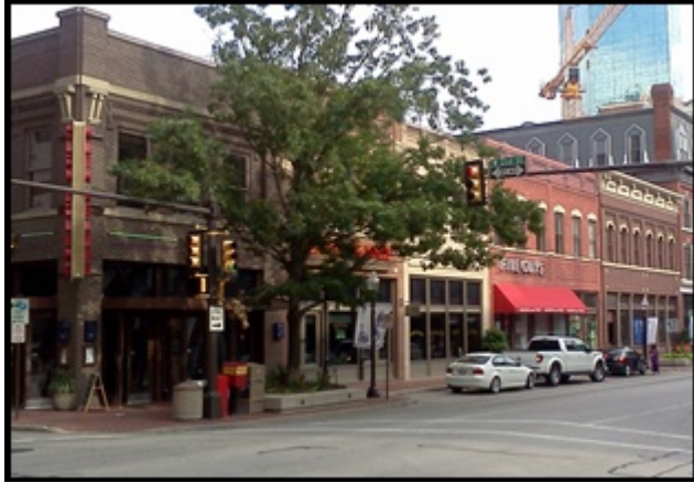
Acceptable change in façade
