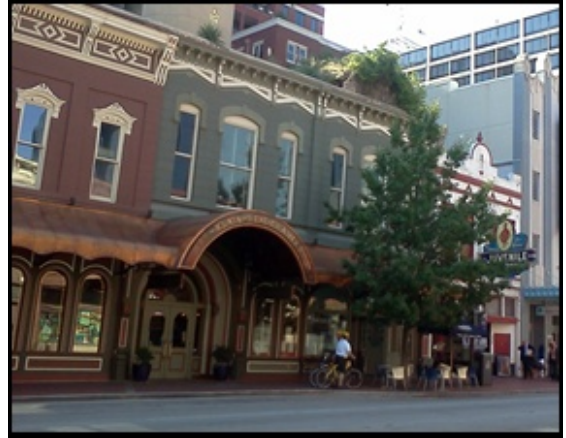
Acceptable change in façade
