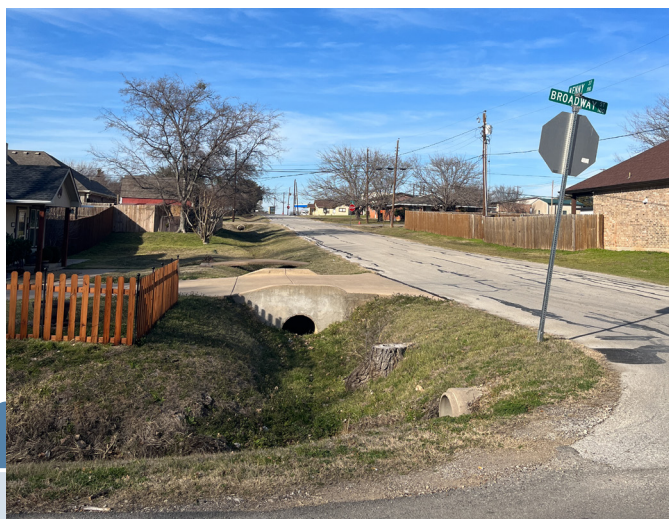
Stormwater infrastructure on a residential street.
