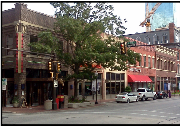
Acceptable change in façade
