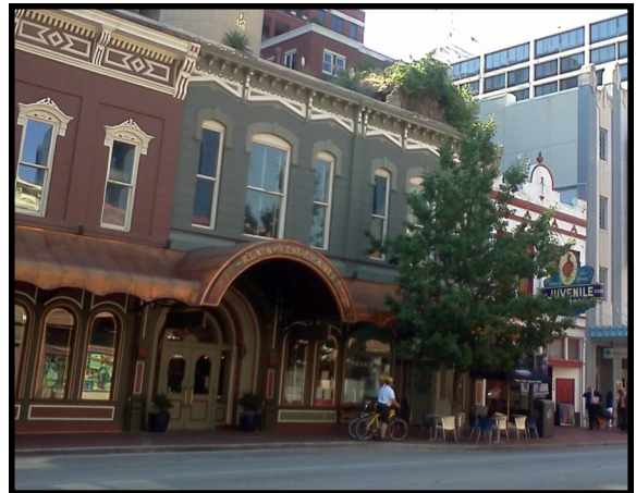
Acceptable change in façade
