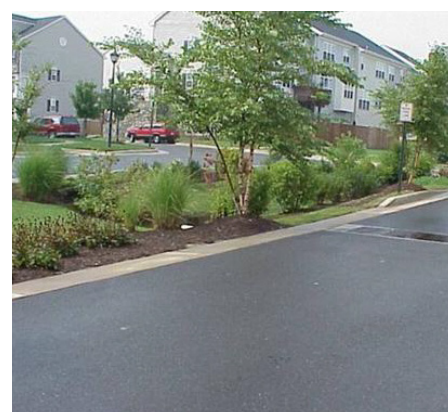
Top image: A bioretention pond in a roadway median; bottom image: a rain garden collects roadway runoff.
