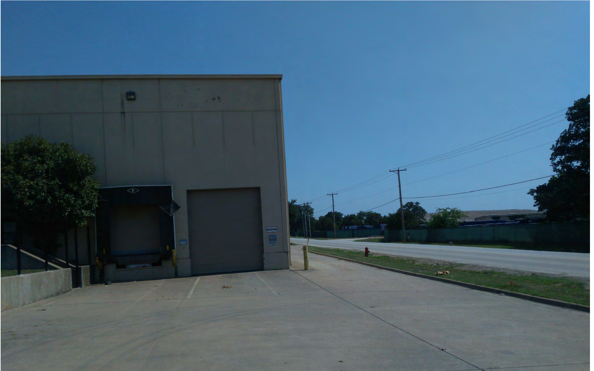
BOA 17-03: additional loading dock off Dick Price Rd
