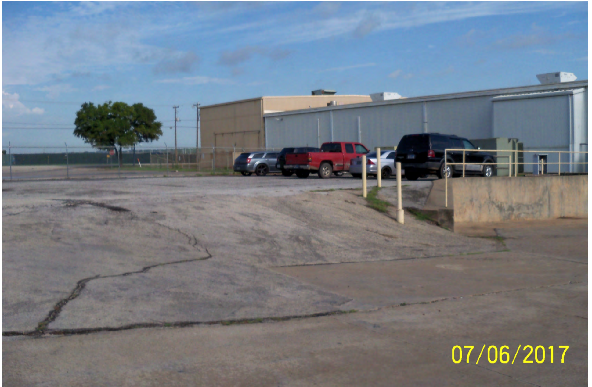
BOA 17-03: looking toward Dick Price from Linda Rd, showing the south side of the main building
