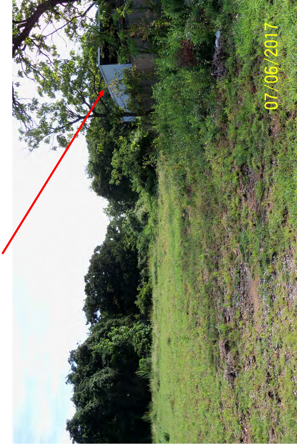
Back of building for BOA 17-05
