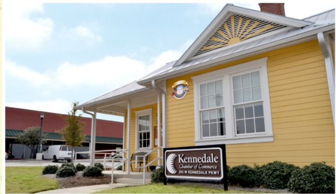
The Kennedale Area Chamber of Commerce, housed in a replica of an original Section House along the rail line that helped establish Kennedale, serves as the anchor of TownCenter.
