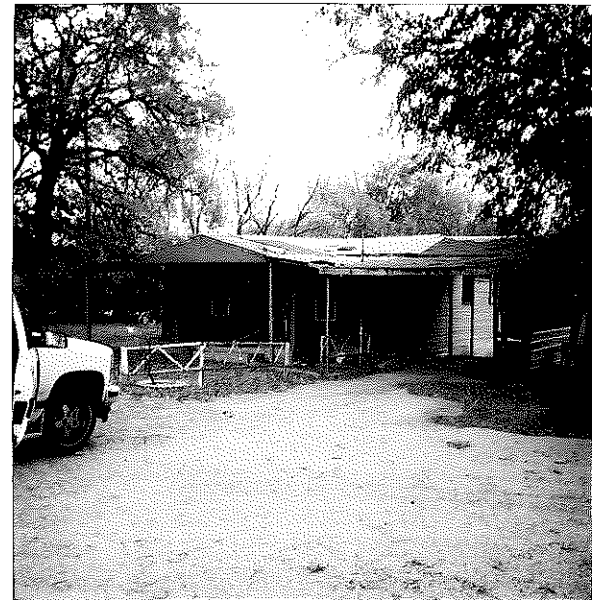
DEMOLD 537 W. MANFIELD Hwy (EMLE EQUIPMENT Co.)
