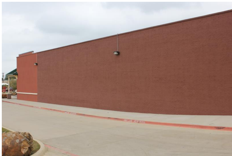
Figure 6. Not permitted: Blank wall is longer than 60 feet, and no articulation is provided along the façade.
