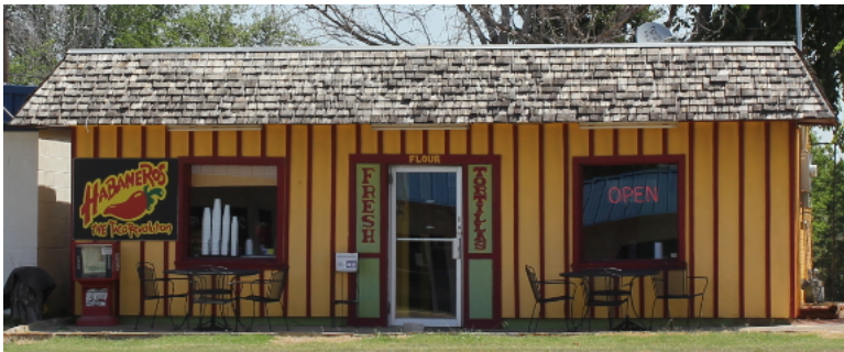
Not permitted: façade with approximately 10% glazing on ground floor
