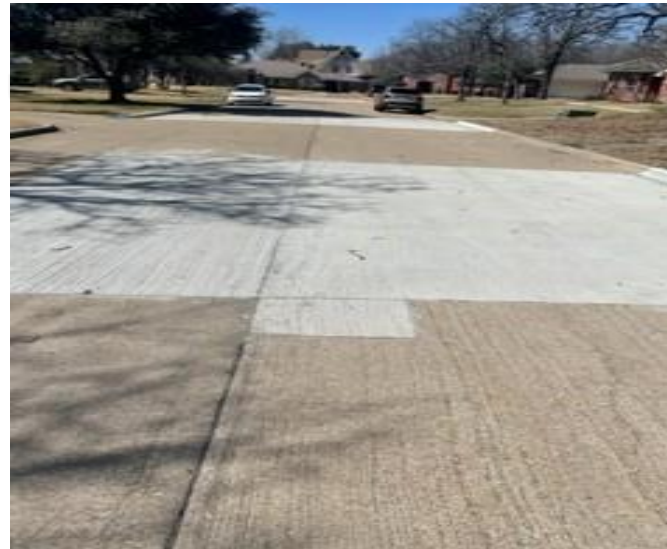
Cross Creek After
